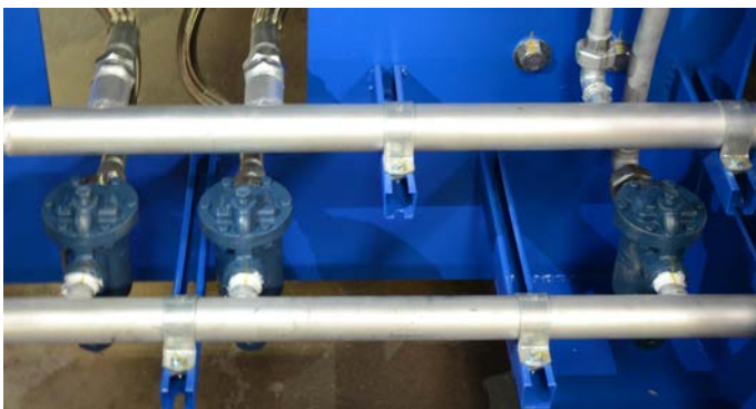
Integrated steam traps for each chamber of the chest
